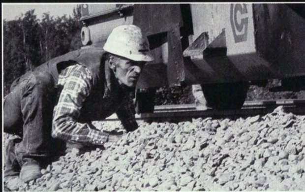
Jim Hubbs, extra gang foreman, oversees an electromatic tamper, a special maintenance device that packs the ballast between rail ties and balances and levels the track.
