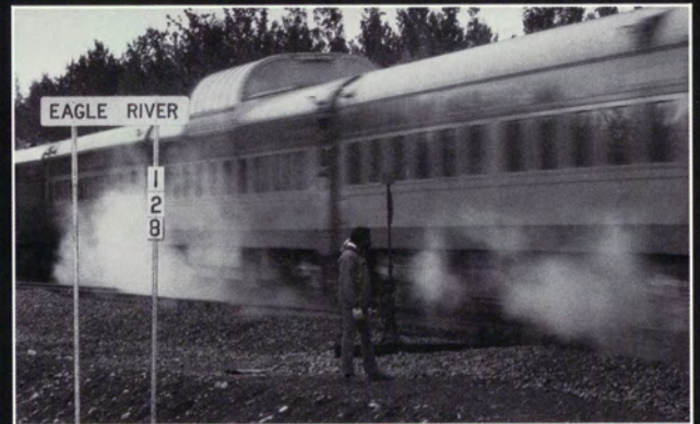
Construction of a 6,201-foot siding at Eagle River provides an intermediate meeting point for opposing train traffic in the railroad's highest traffic density area.
