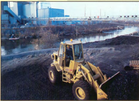
Coal-fired steam boilers at the Fairbanks Municipal Utility System provided 118 million kilowatt-hours of electricity and 146 million pounds of steam for steam heat to Fairbanks area residents in 1987. All of the coal for the facility is shipped via the Alaska Railroad and stockpiled in the MUS yard.
