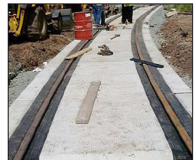
Rail flangeways filled with rubber.
