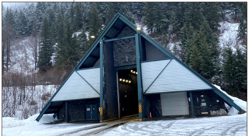
The west entrance to the Anton Anderson Memorial Tunnel, February 2021.
