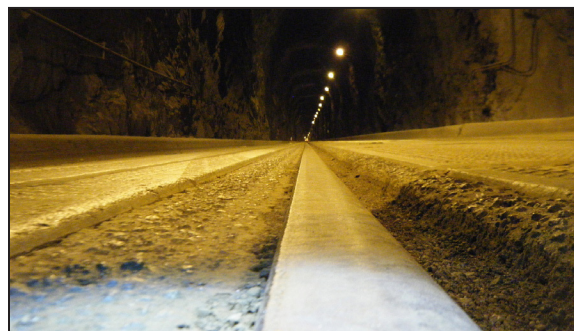
Rail flangeways filled with asphalt.
