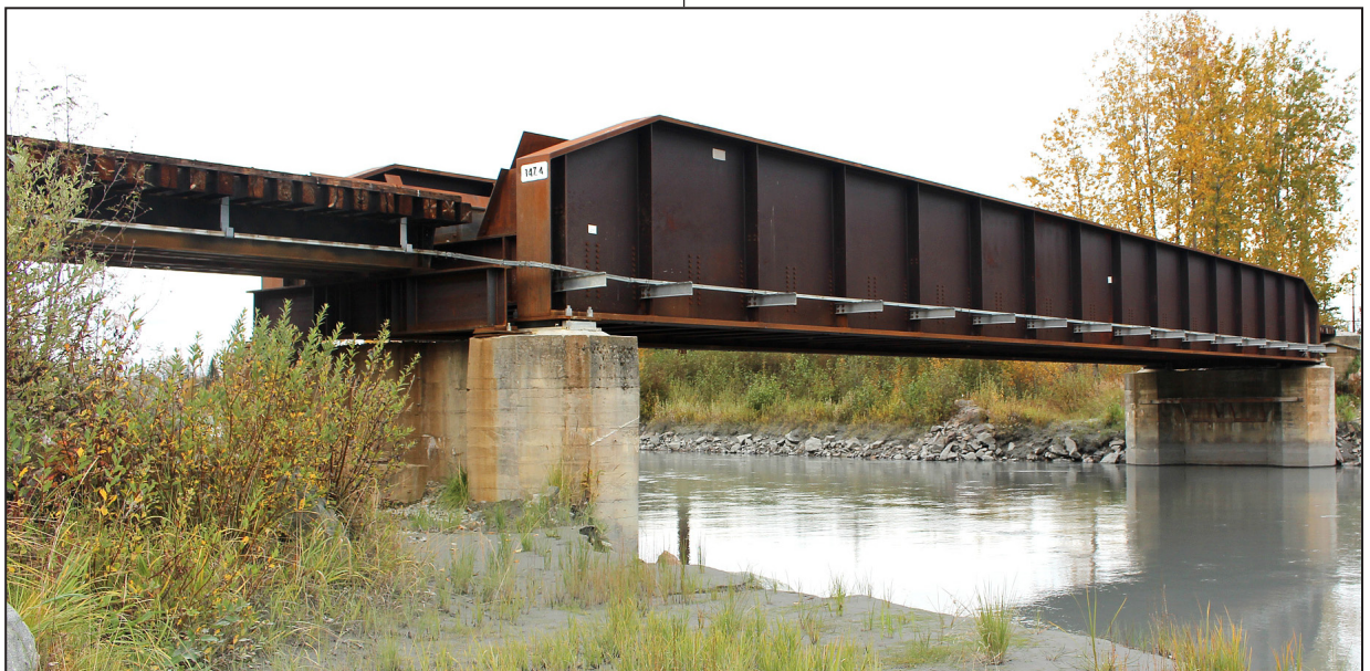
Bridge 147.4 over the Matanuska Flood Channel.
