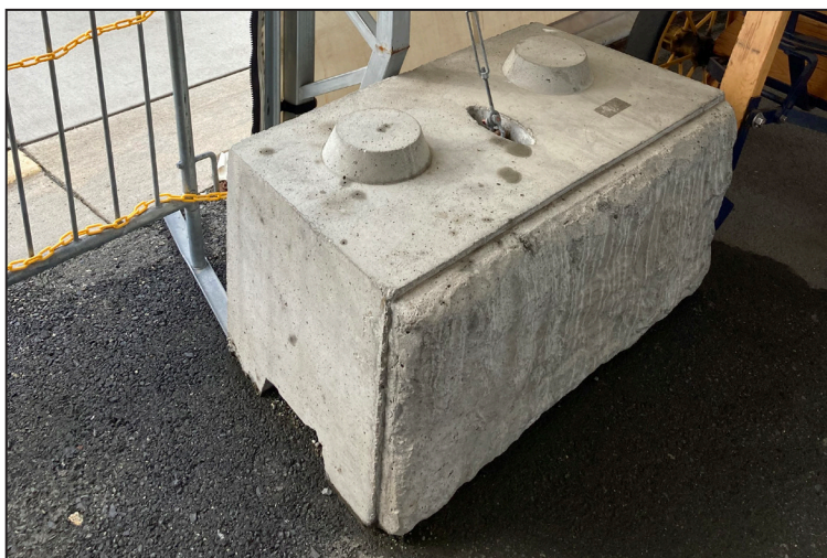
Concrete tie-down blocks anchor the Anchorage depot baggage shelter.
