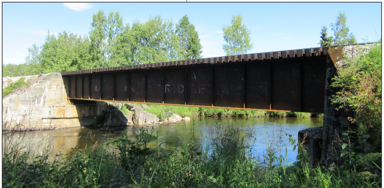
Bridge 190.5 crosses Little Willow Creek just north of Willow.
