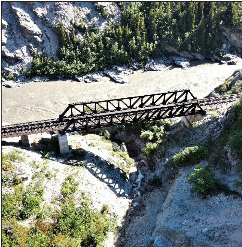
Bridge 354 crosses Bison Gulch along the banks of the Nenana River.
