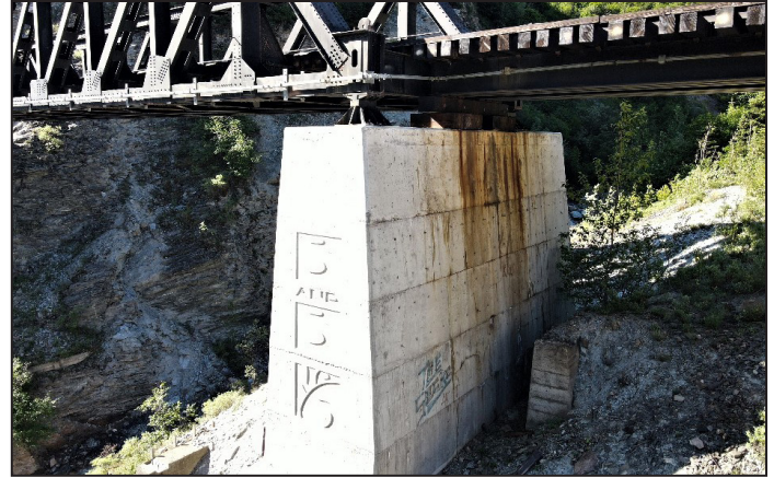
Existing piers will be reused to support the new bridge.
