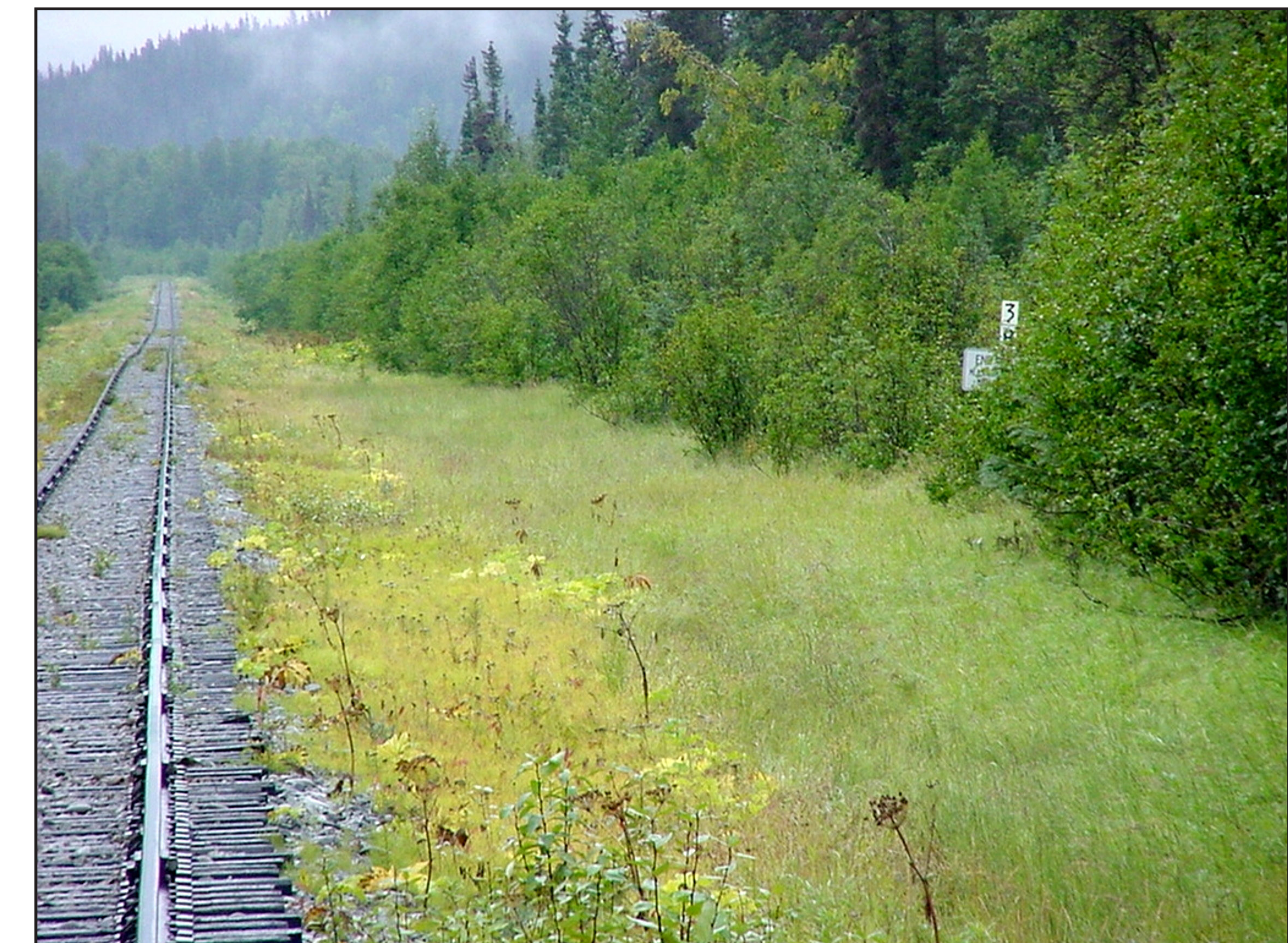
Obscured signs and infrastructure pose safety concerns.
