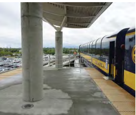
Level Platform Loading at Airport Depot
