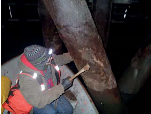
Cleaning and Inspecting Batter Piles
