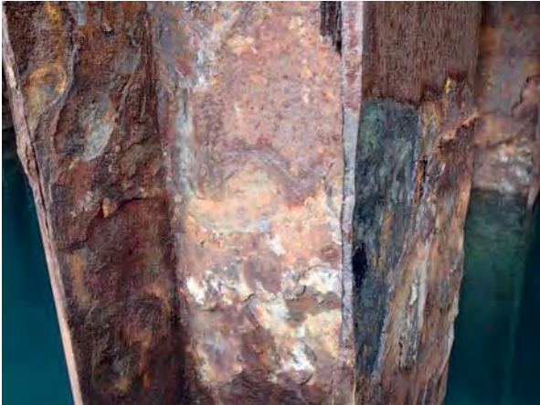
Corrosion of H Piling in the Splash Zone
