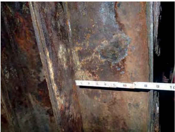
Corrosion of H Piling in the Splash Zone
