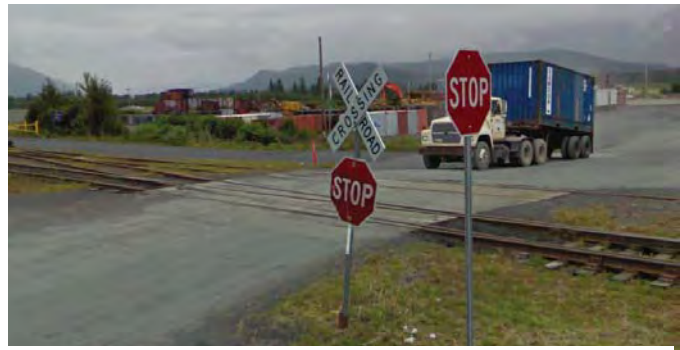
Passenger Dock Tracks, Port Avenue At-Grade Crossing
