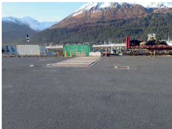
Slot in Deck for Baggage Handling
