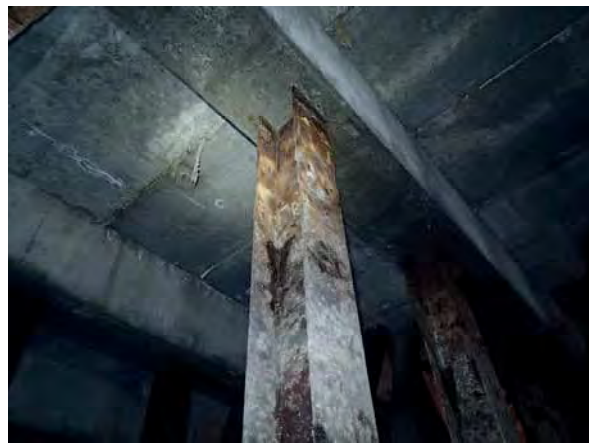
Bottom of Precast Deck Panels
