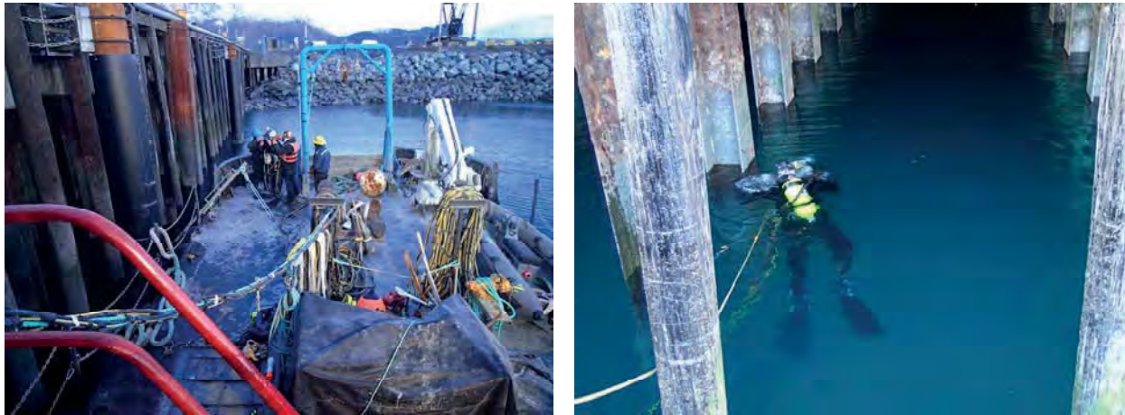
Surface Supplied Diving Operations with Helmet Mounted Video Camera
