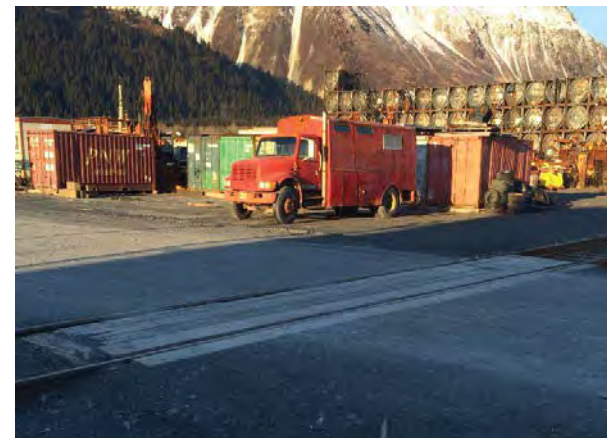
Wood Tie At-Grade Crossing at Port Avenue
