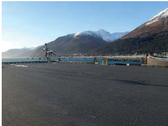
Deck with Asphalt Overlay
