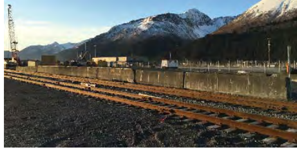
Side Loading Ramp Along Freight Dock Track No. 2
