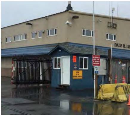
Guard Shack and Gate
