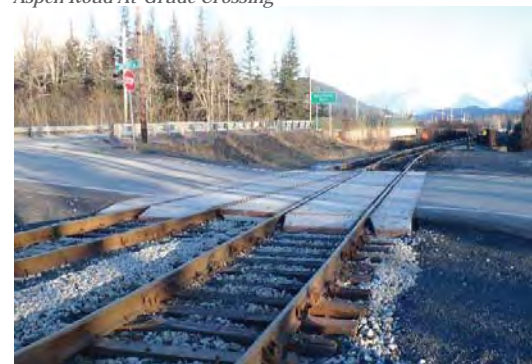
Airport Road At-Grade Crossing
