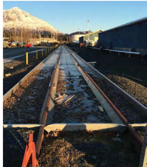
Shoreside Petroleum Spur, Containment Pans
