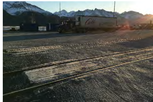
Wood Tie At-Grade Crossing North of Freight Dock
