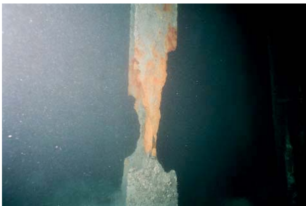
Underwater Photo Bent 10 Pile 11
