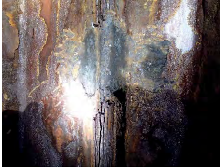
Sheet Pile Interlock at Abutment
