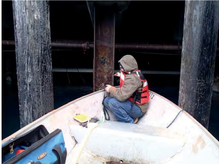
Inspecting Piling from a Skiff
