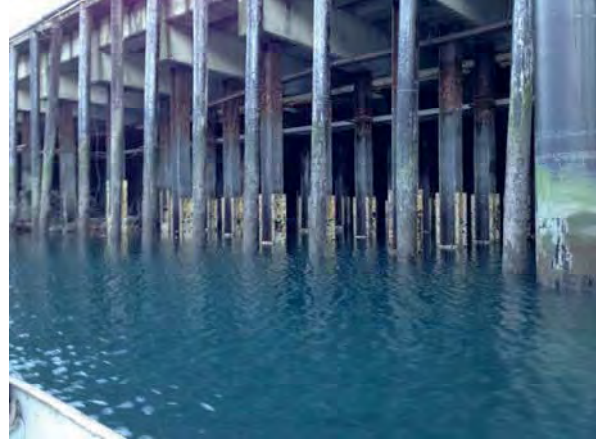
Pile Repair Clamps
