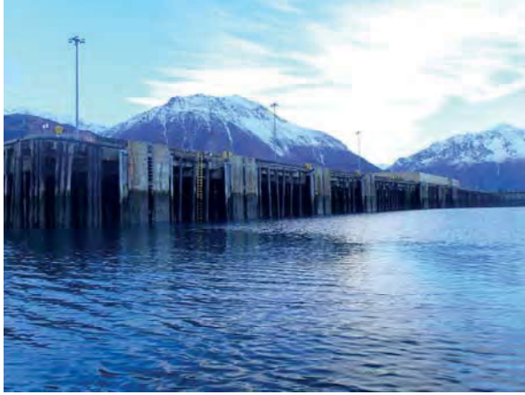
Main Fender at East Side of Dock
