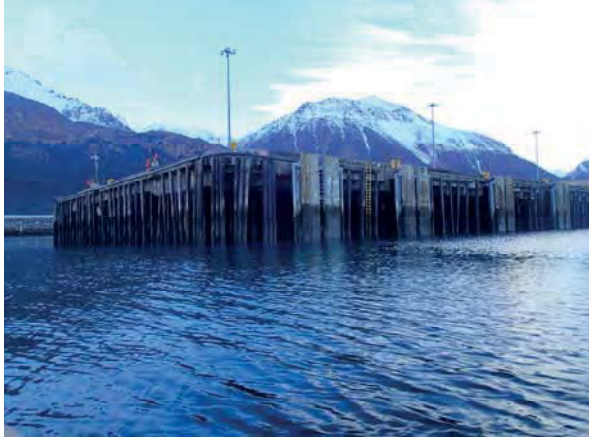
Fender Piles at End of Dock
