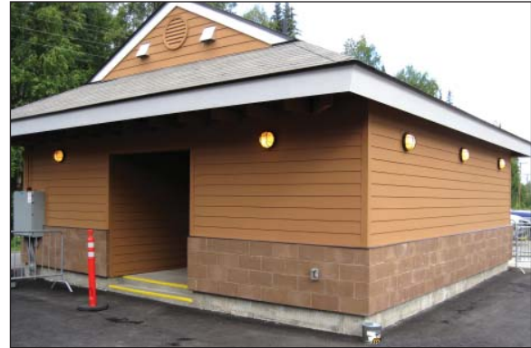
The Talkeetna restroom facility nears completion in 2010.
