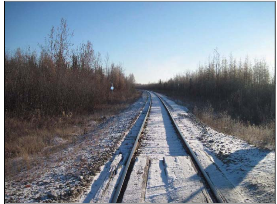
SE View at Rentals St. Crossing
