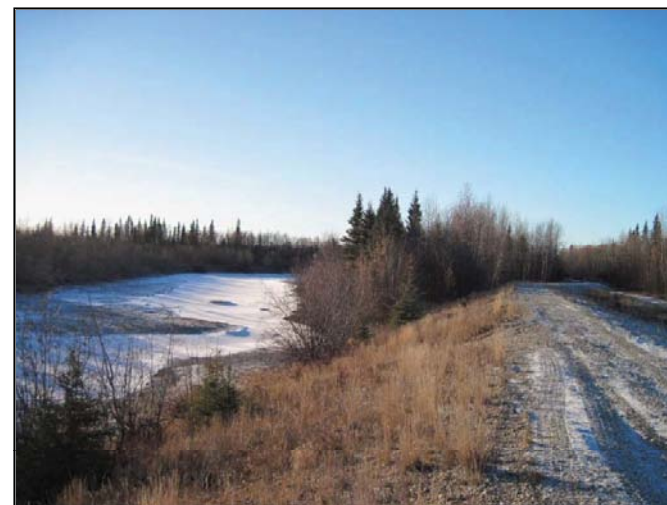
SW view on Levee at Tanana River
