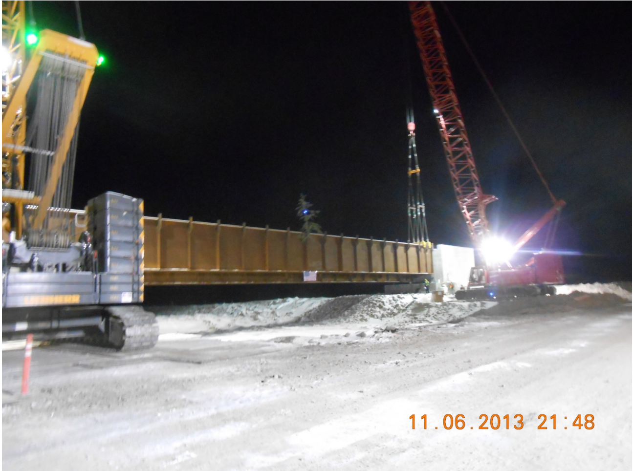
Last bridge girder erected
