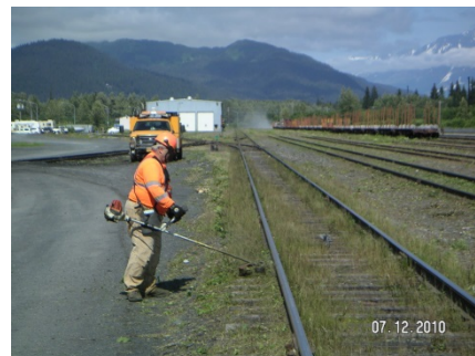
Mechanical control in Seward Yard is not effective in meeting vegetation management requirements.
