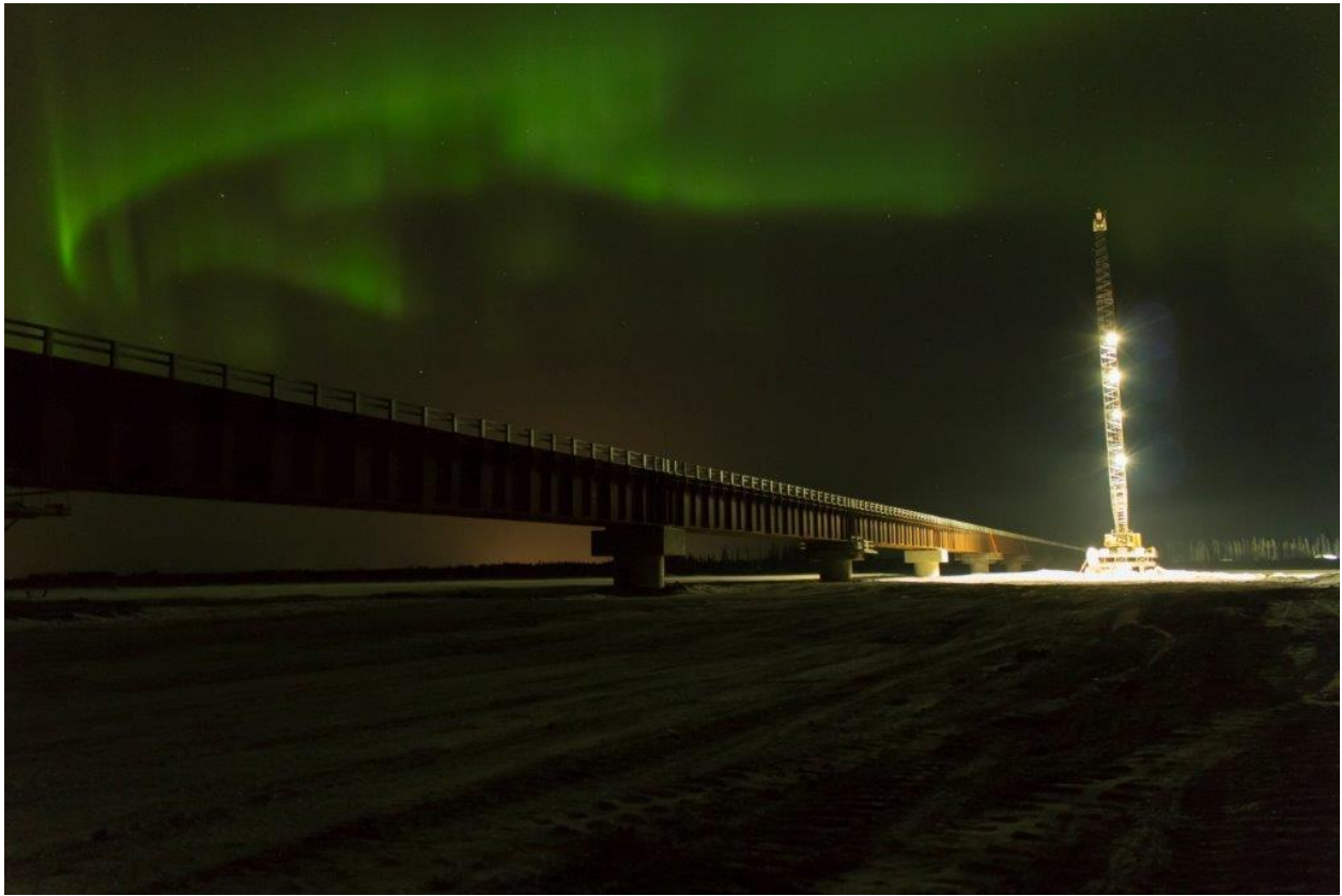
Last bridge girder erected
