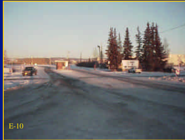
South Gate Crossing, Ft. Wainright
