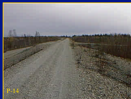
View along Levee at Spur Dike
