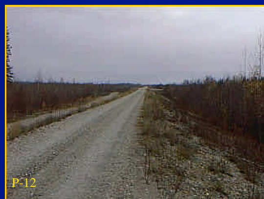
Begin Alignment on Levee
