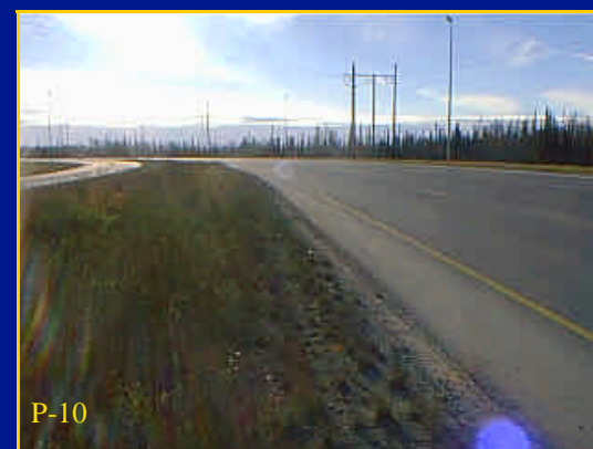
End Median Use, Traverse to Levee
