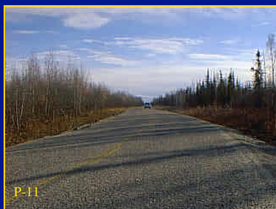
Cartwright Road Crossing
