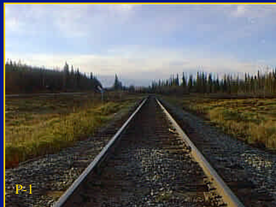
Beginning of Realignment
