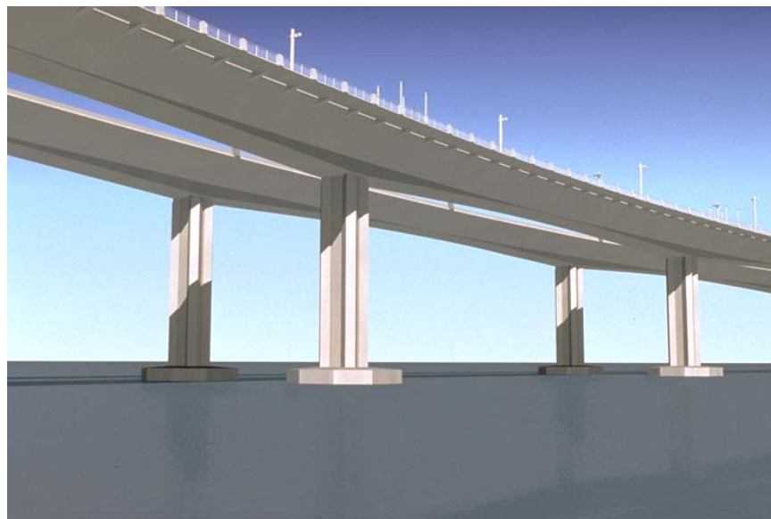
Figure 3.33. San Francisco-Oakland Bay Bridge
