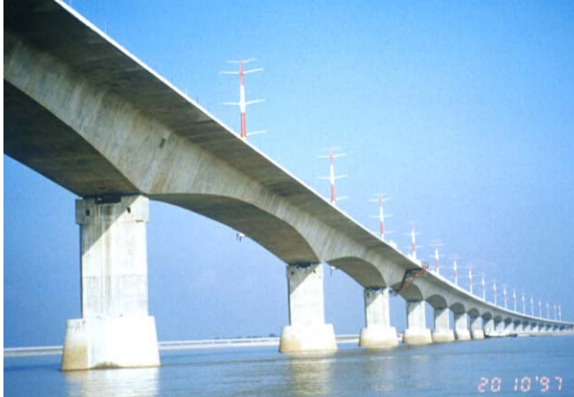
Figure 3.34. Jamuna River Bridge
