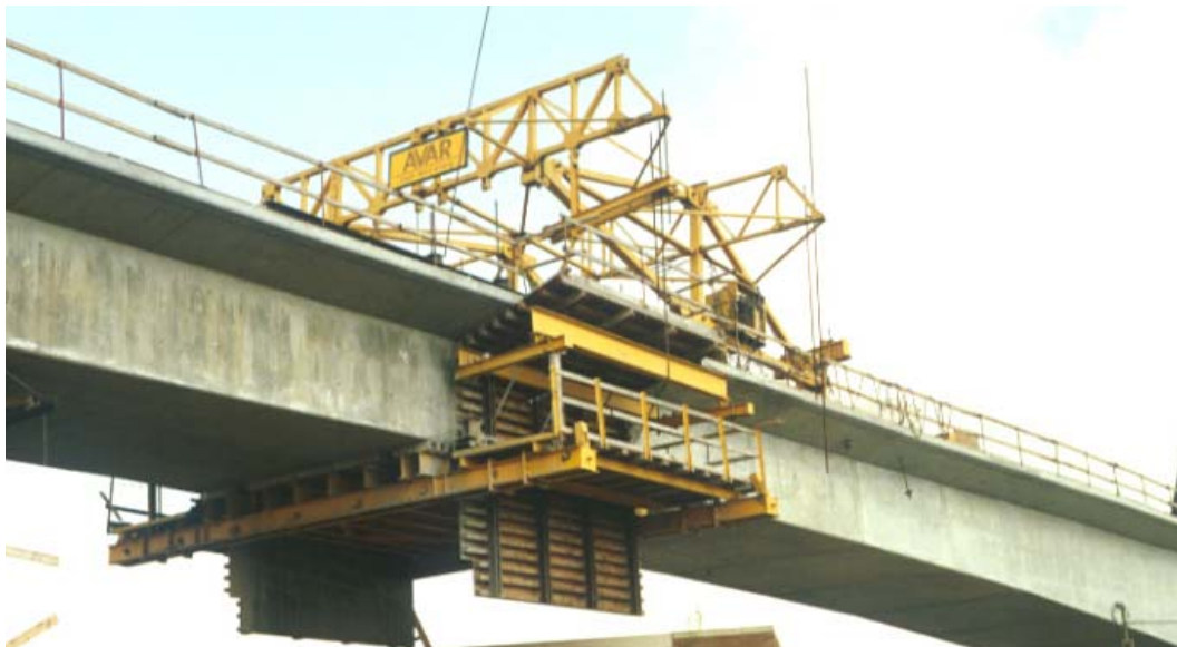
Figure 3.17. Casting of Closure Segment (Kramer-Rosecrans Bridge)
