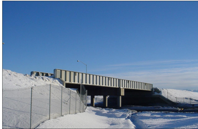
Example of a grade-separated rail crossing (“Rail over Road”) over Dimond Boulevard in south Anchorage
