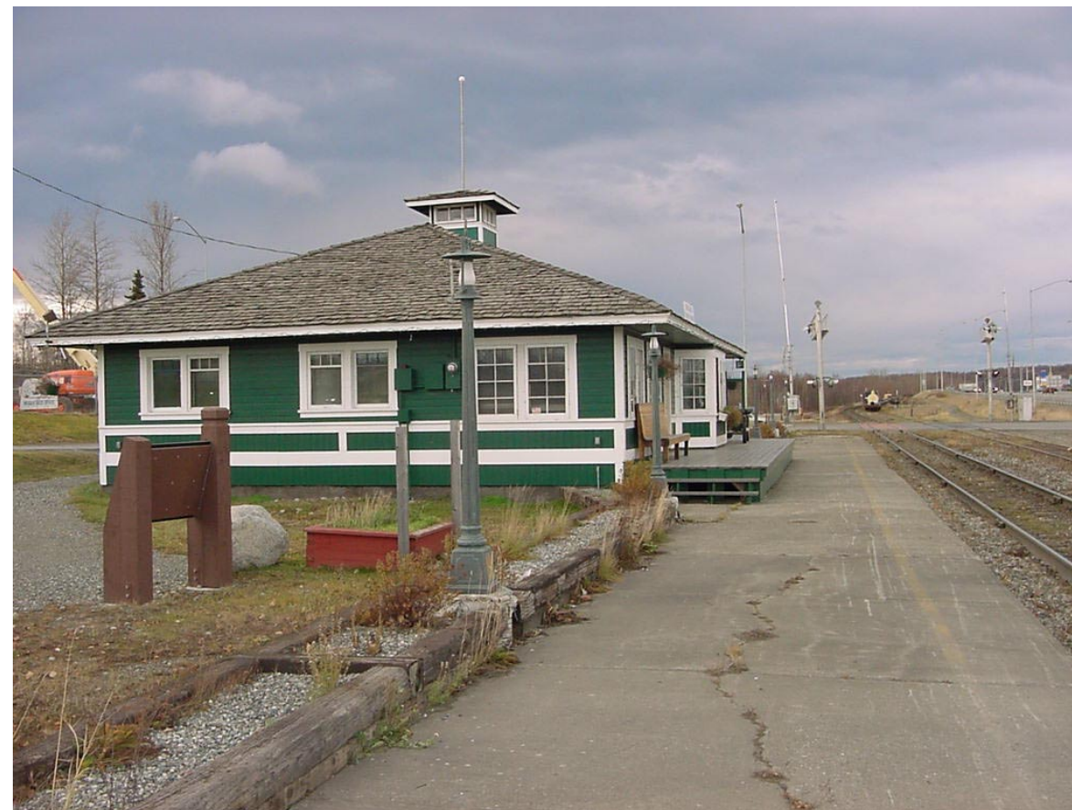
The Wasilla Historic Depot & existing railroad platform and tracks are located immediately south of the Parks Highway and east of the Knik-Goose Bay Road
