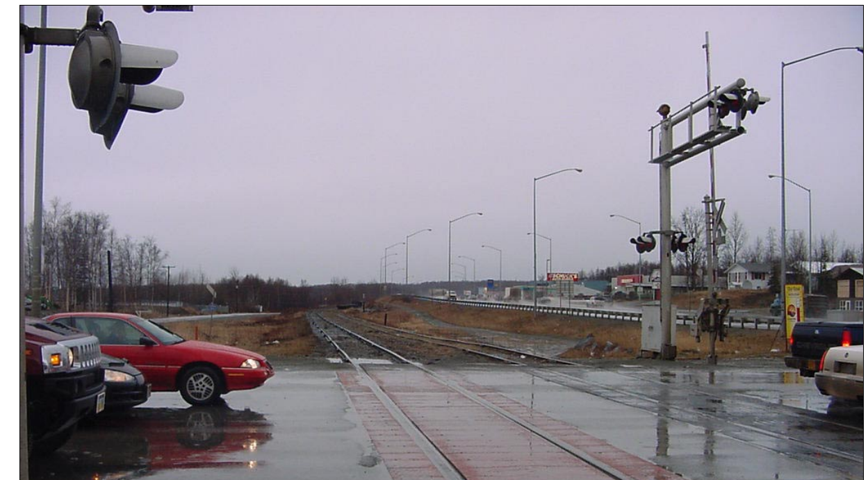
Knik-Goose Bay Road Existing At-grade Crossing in Wasilla, Alaska
